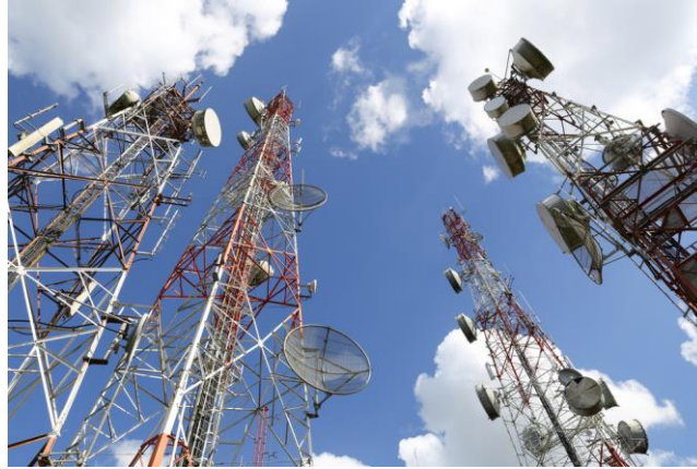
Figure 5: Very congested site example
